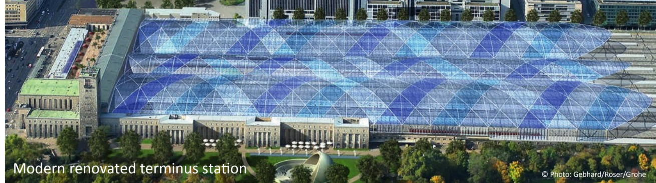
Modern renovated terminus station
